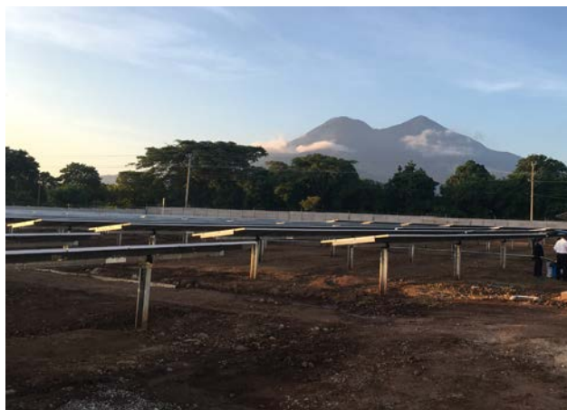
Single-axis solar PV tracking system in Central America (Photo credit: Laird Reed)
